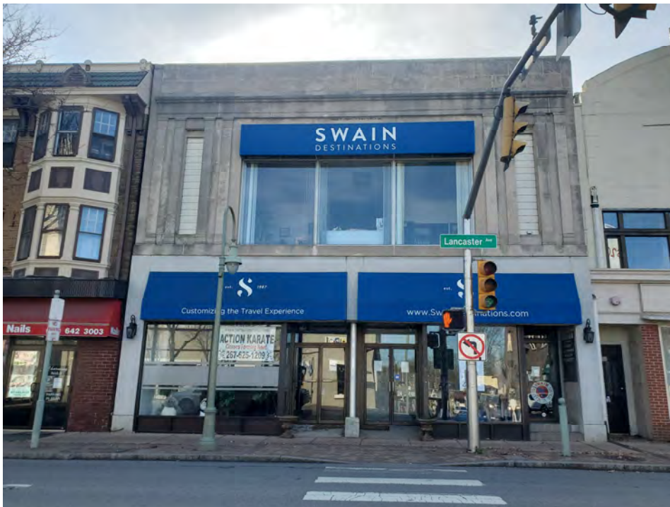
Photo 10: View of the Site.
