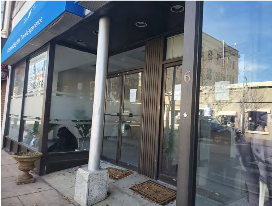
Photo 9: View of the Front Entrance to the Site Building, on the Northern Side of the Site.
