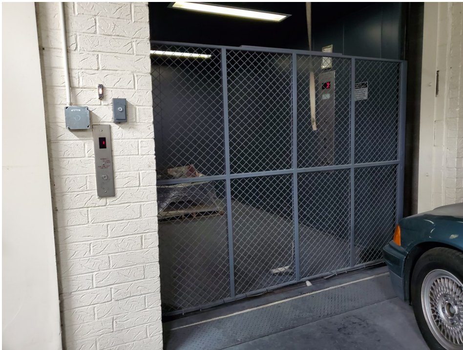
Photo 8: View of the Elevator Inside the Garage at the Site.
