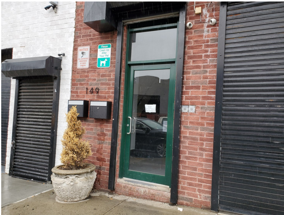
Photo 6: View of the Front Entrance to the Site Building.
